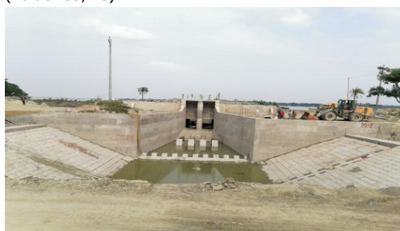
Figure 3-26: Bank Protection with Pitching Works (Polder 39/2C)
