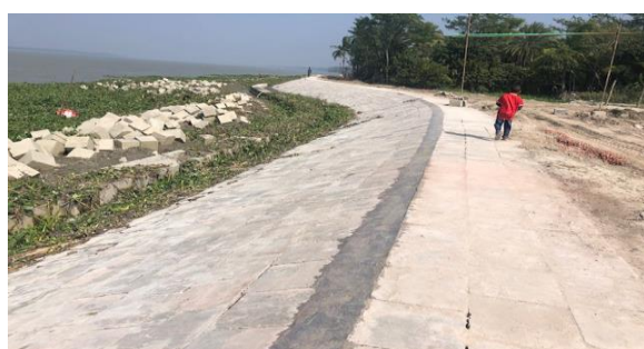
Figure 3-26: Bank Protection with Pitching Works (Polder 39/2C)
