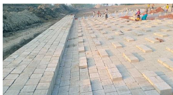
Figure 3-27: Ongoing Slope Protection Works (Polder 40/2), Barguna
